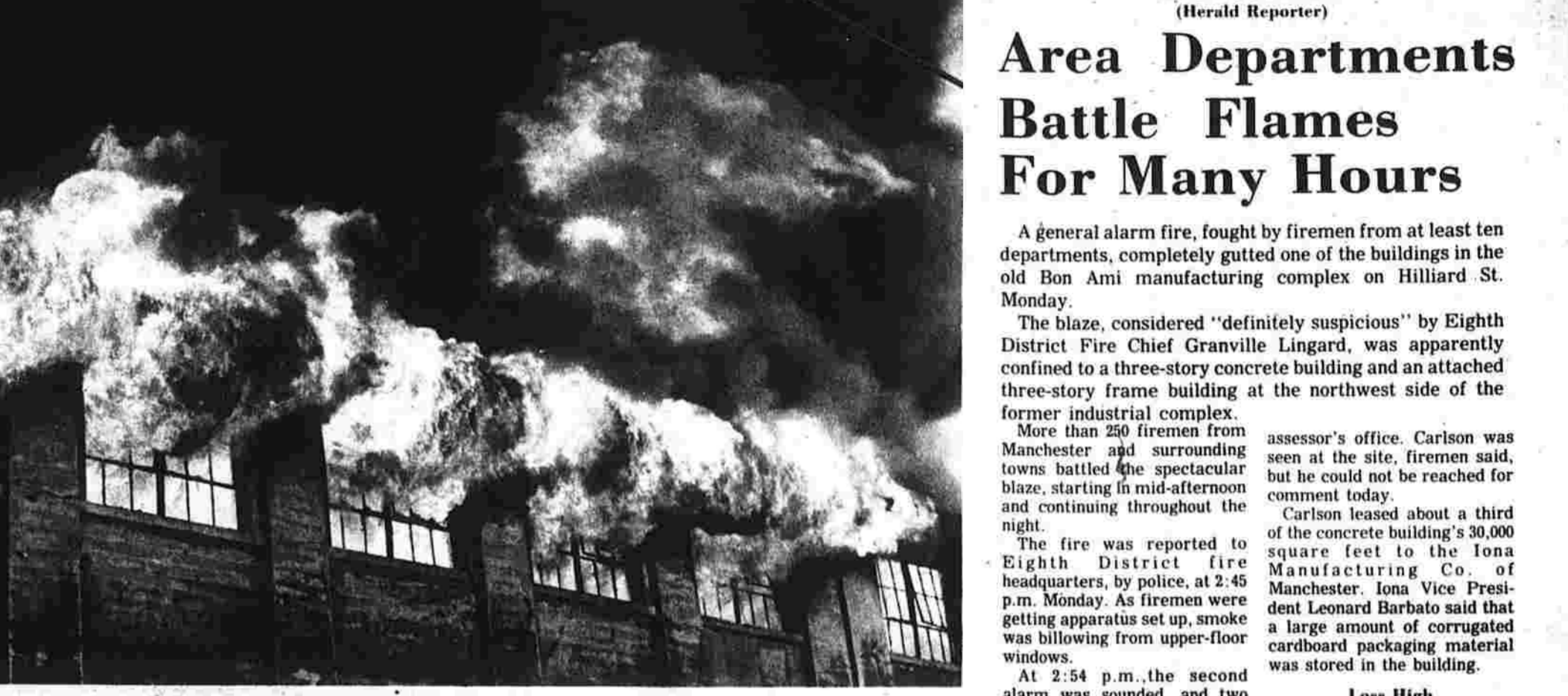
Flames Belching From Old Factory Windows The extent of the old Bon Ami Complex fire in Manchester yesterday afternoon is graphically shown in this photograph of the blaze which was brought under control about six hours after it was reported through the combined efforts of several firefighting units. (Herald photo by Pinto)
