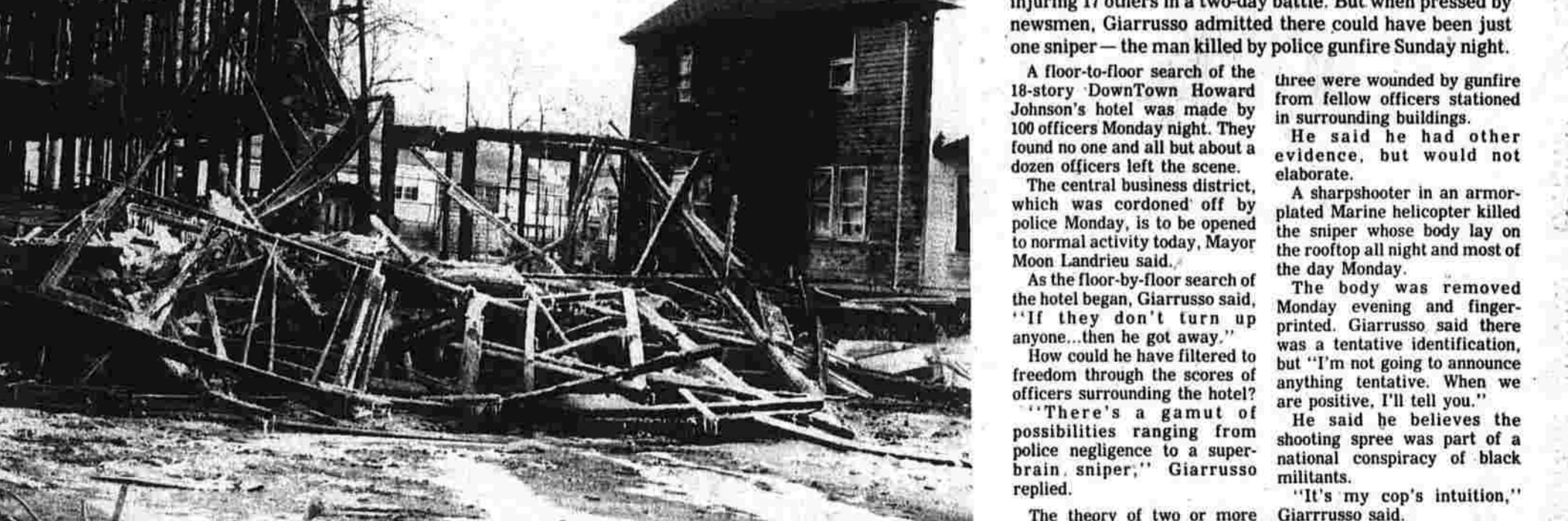
The Remains Of An Intense Fire The limp, charred frame of a building under construction on W. Middle Tpke., is all that was left after an early morning fire of "suspicious origin" gutted the nearby completed building and caused extensive damage to the house next door owned by Tony Vernali. The destroyed building was being constructed by Nicholas Jackson by the Hohenbach Company of Center St. The owner set the value of the building at $60,000. The damage to the Vernali home has not yet been estimated. (Herald photo by Pinto)
